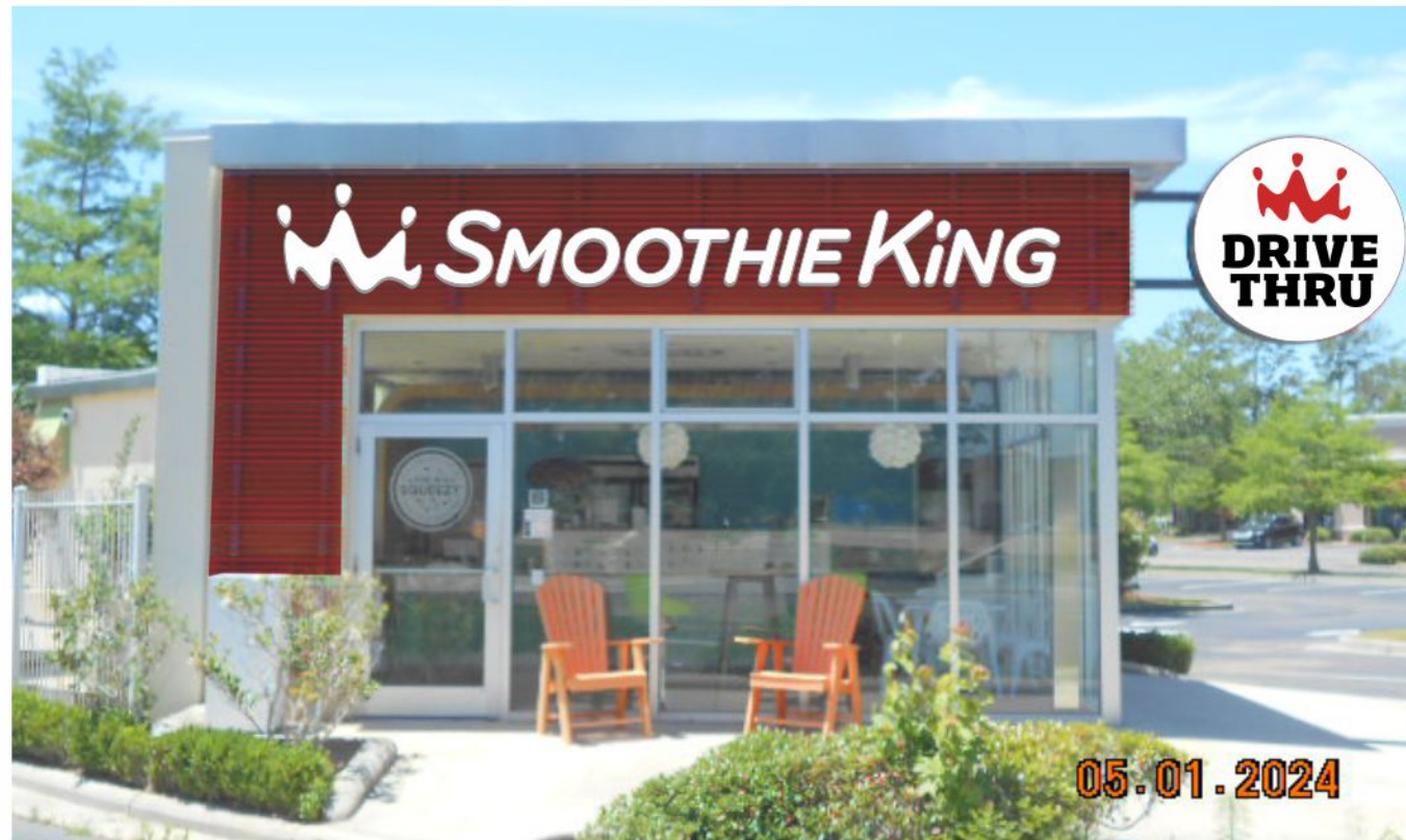
Tube grid wall is to be painted SW 7593 Rustic Red by others.
