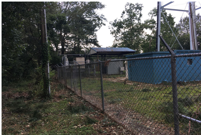
Photo Depicts damaged Barbed wire.
