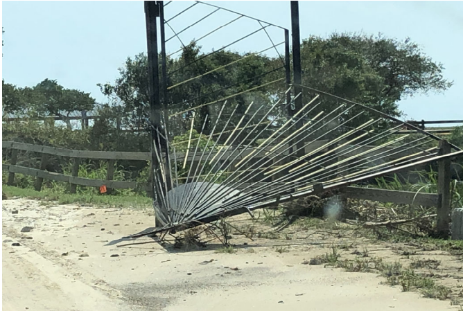
Photo Depicts Ornamental Gate damage.
