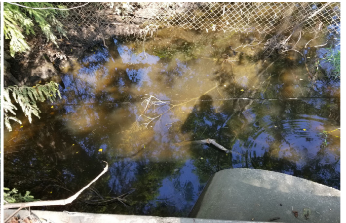
Photo Depicts fence crossing canal.
