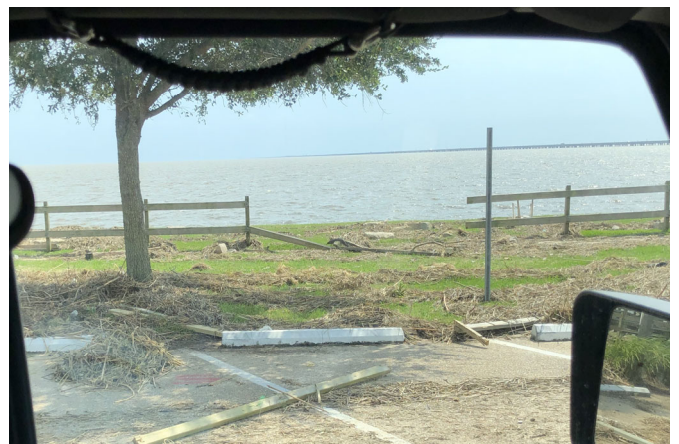
Photo Depicts wooden fence damage.
