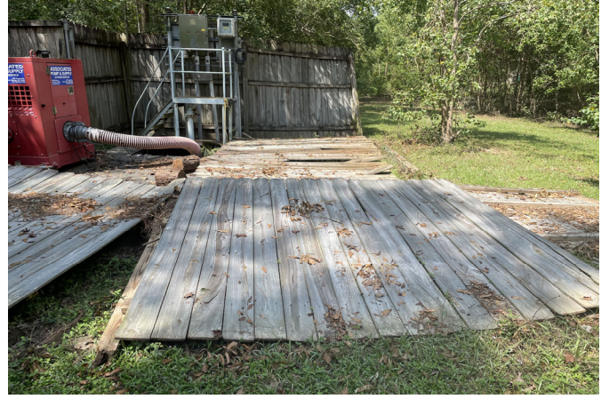
Photo Depicts damaged wooden fence.
