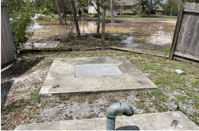
Photo Depicts wooden fence missing sections and damaged.
