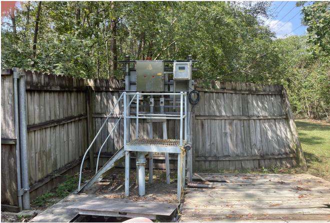
Photo Depicts another view of damaged wooden fence.
