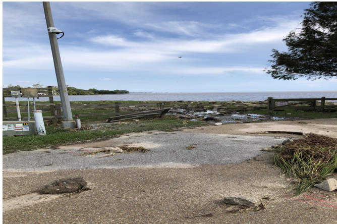
Photo Depicts wooden fence damage.
