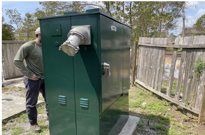
Photo Depicts Fence missing boards and leaning.
