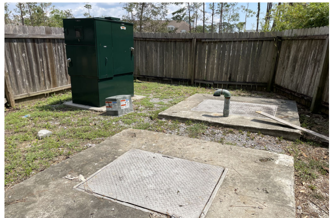
Photo Depicts saggin fence framing and leaning posts.
