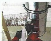
Duct Sealing
